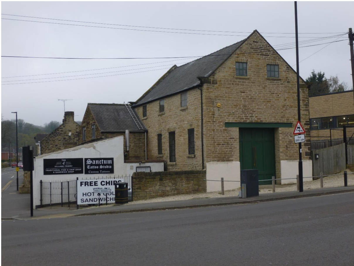
The former Corn Mill, on the junction of The Common and Mill Road, Ecclesfield.
