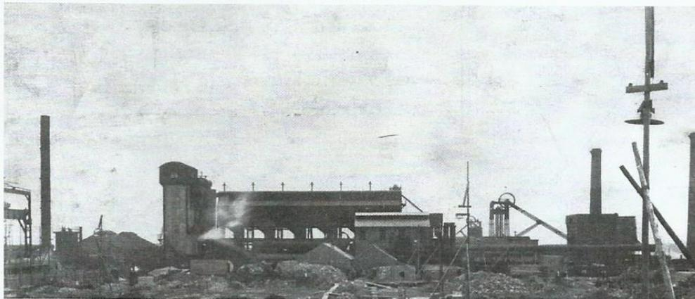
This photograph shows Langwith Bye-Products Plant. 1916 The colliery is to the rear right. The gas was burnt off from the six chimneys above the retorts.
