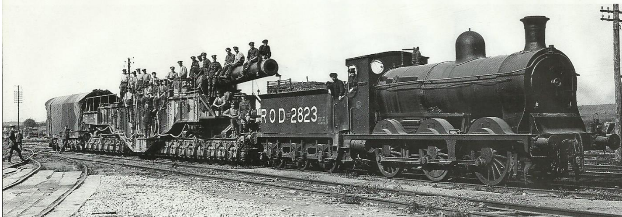
The "Boche Buster": This enormous 14-inch naval gun, mounted on 16 axles, was one of two shipped from Britain to France to bombard the German defences. It is pictured on August 8, 1918 – the day it was demonstrated to King George V at Maroeuil, near Arras. It was later taken back to the UK and was used again in the Second World War, being based on the Elham Valley Line in Kent. Although part of Britain's Railway Operating Division fleet, loco No. 2823 is an ex-Belgian State Railway Type 30. IMPERIAL WAR MUSEUM
