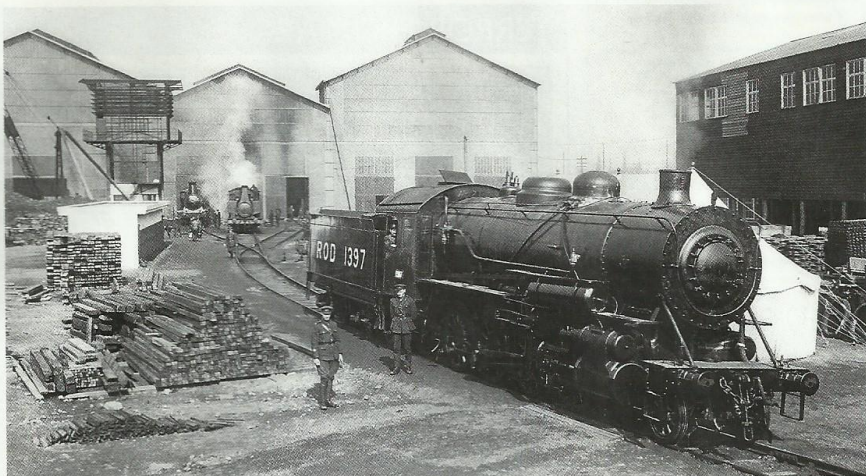
ABOVE: An indication of the scale of the British and Allied railway operation in northern France can be gained from the size of the Railway Operating Division's workshops at St Etienne-du-Rouvray. Baldwin 2-8-0 No. 1397 has just been assembled and is undergoing steam tests before entering service. IMPERIAL WAR MUSEUM
