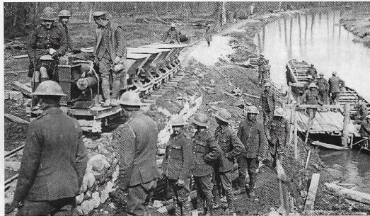
Royal Artillery men at work on a field railway alongside the River Scarpe at Blangy, France, in April 1917. IMPERIAL WAR MUSEUM
