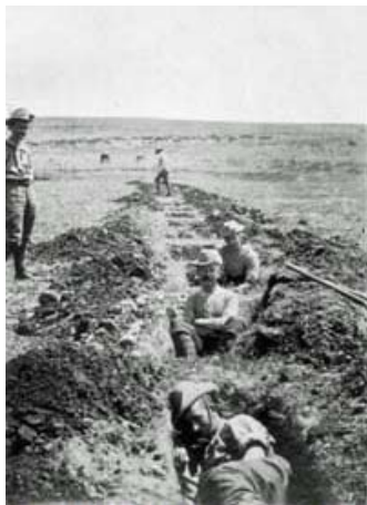
Digging slit trenches against air attack
