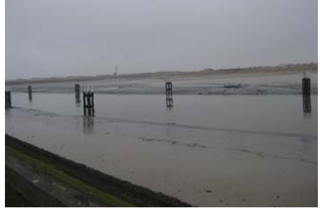
View across Ijzer from West bank
