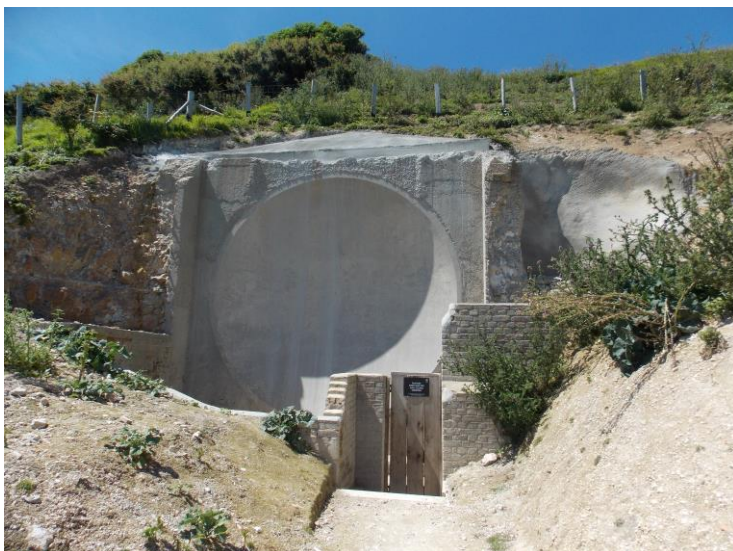
One of the 15 foot diameter sound mirrors at Fan Bay near Dover Photo: Tim Keenan
