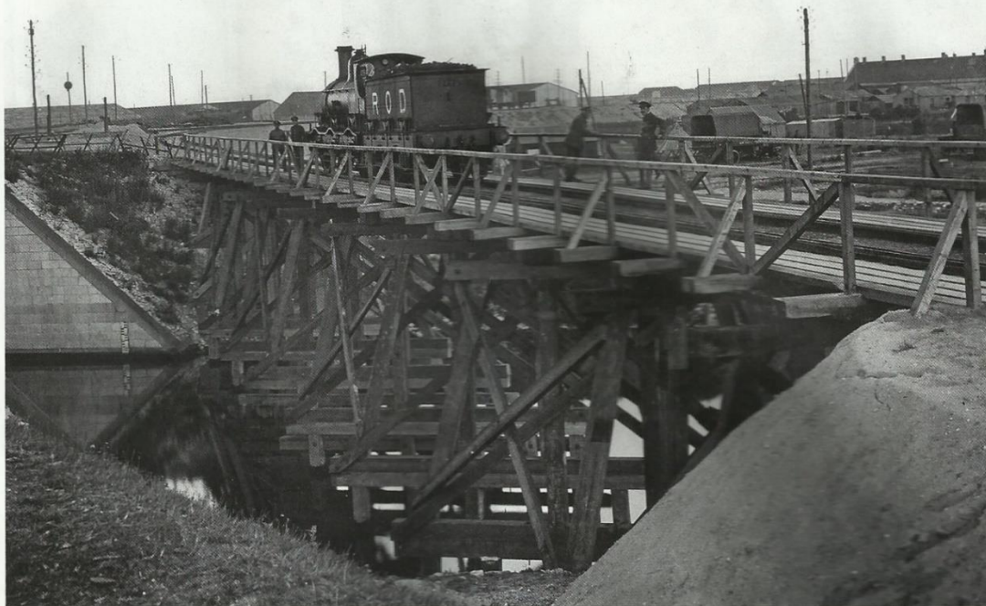
A Midland Railway 0-6-0, ROD No. 2723, crosses a substantial wooden trestle bridge built by the Royal Engineers to re-connect the docks and marshalling yard at Dunkirk, WWI
