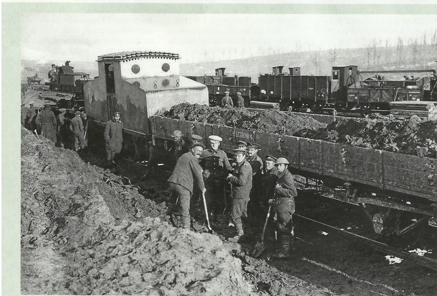
LEFT: This unusual photograph shows one of the few non-steam examples of ROD motive power.
