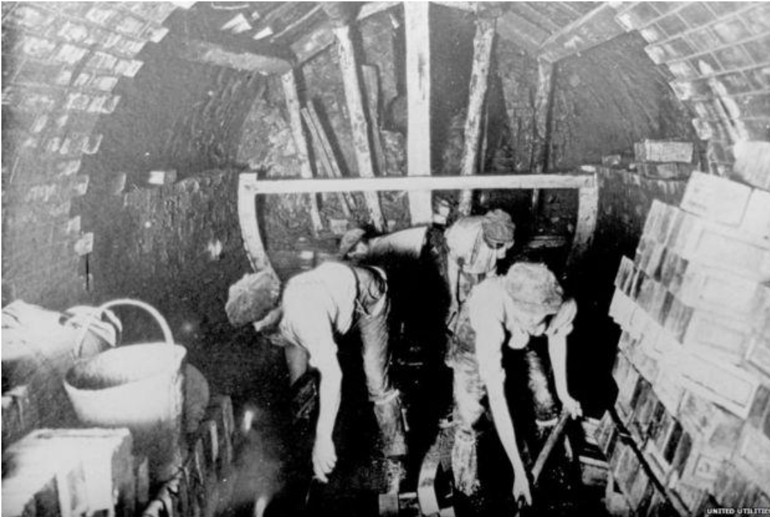
Work on Manchester Corporation's drainage system
