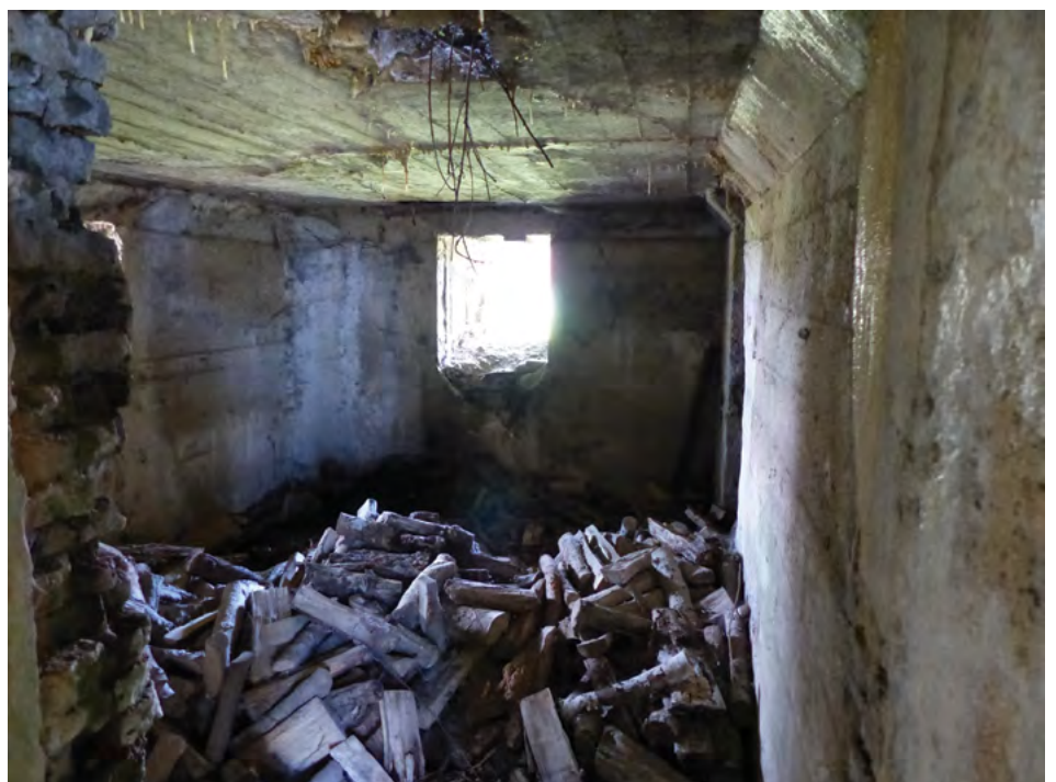
Interior of Bunker at Gournier Farm
