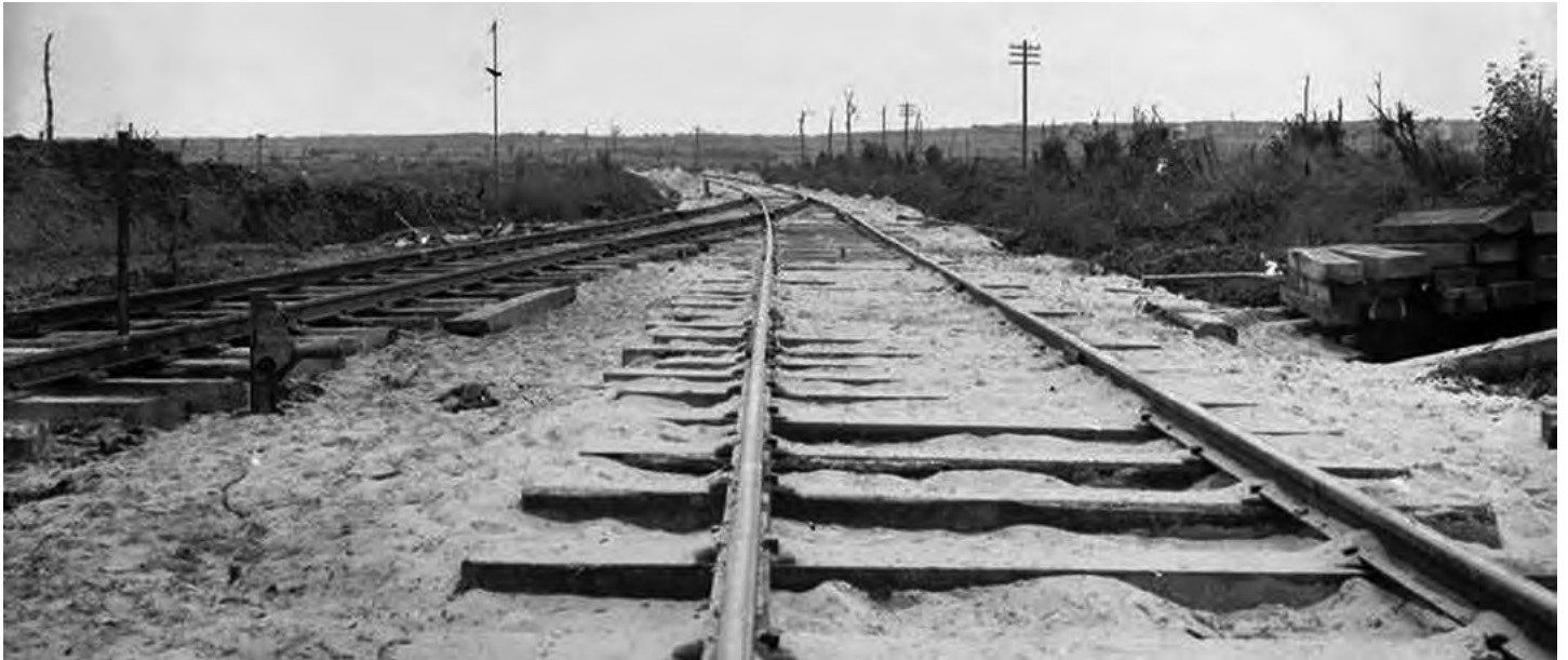
The view along the Ypres–Roulers railway line from Zonnebeke Station on 10 October 1918 photographed after a week of intensive engineering work. The early stages of the tour follow the line of the track as it ascends the Passchendaele Ridge in the distance. Courtesy IWM Q46667
