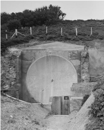
The sound mirror at Fan Bay, Dover, has a diameter of 15ft.
