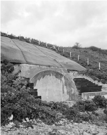
The sound mirror at Fan Bay, Dover, has a diameter of 15ft.
