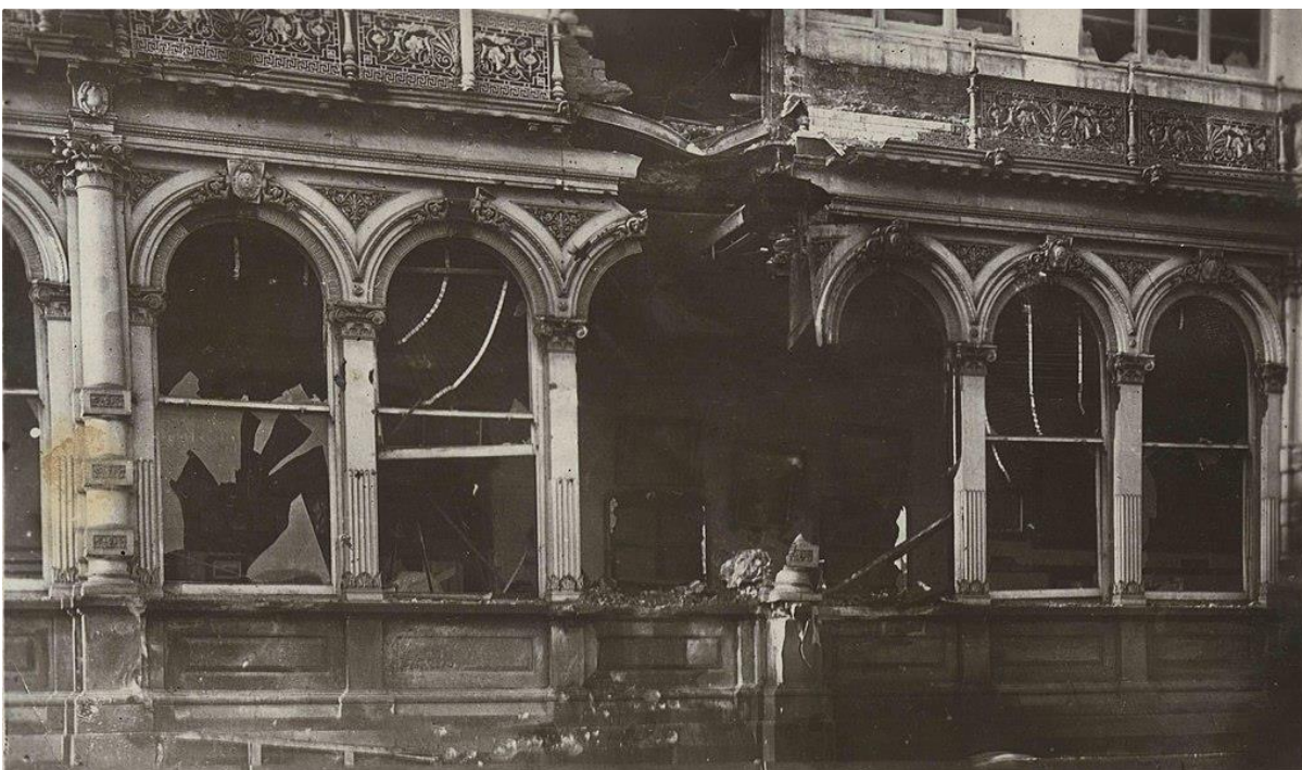
Damage to the Grand Hotel at Scarborough
