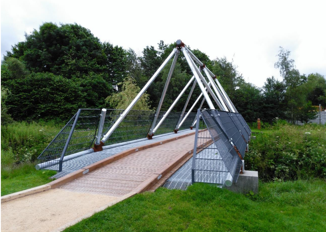
The newly installed Inglis Bridge over the River Lostock. Photograph by Charlie O'Donnell
