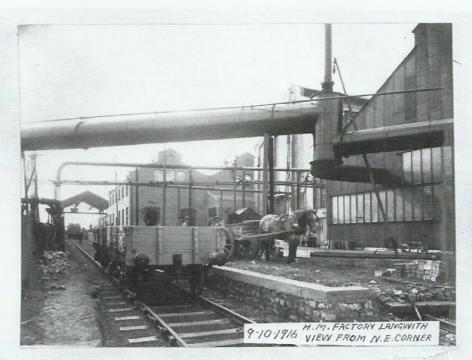
The big pipes bringing the gas from the bye products plant into the gas cleaning plant. The engine house is behind the horse and cart to the right,
