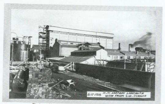
The tower block where the chemical was made is completed. The smoking chimney to the right is the bye-products plant making the gas for the generators.
