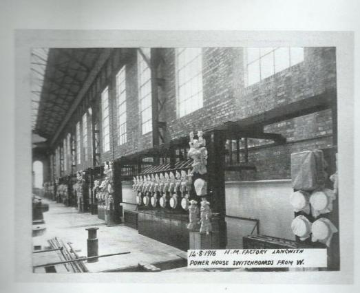
This is a photograph of the switch gear sending the power to the hydrolysis or acid department next door.
