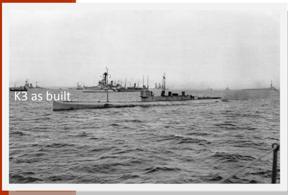
The immediate problem facing this idea was that the normal speed of the battle fleet in 1916 was 21 knots (about 24mph). Any vessel keeping company with the fleet would need 2/3 knots above this to enable them to manoeuvre and keep station within the fleet and to move ahead towards the enemy before diving and closing to attack at their lower submerged speed. A fleet submarine would therefore require a surface speed of about 24 knots (27.5mph).
