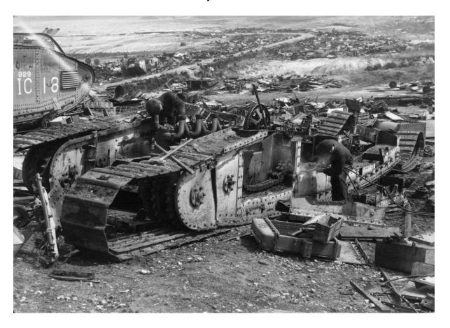
Scrapping of a Gun Carrier Mark I, with a Mark IX and Mark V\* in the background, likely taken at the Steelbreaking and Dismantling Company of Chesterfield. Photo from the Evening Standard
