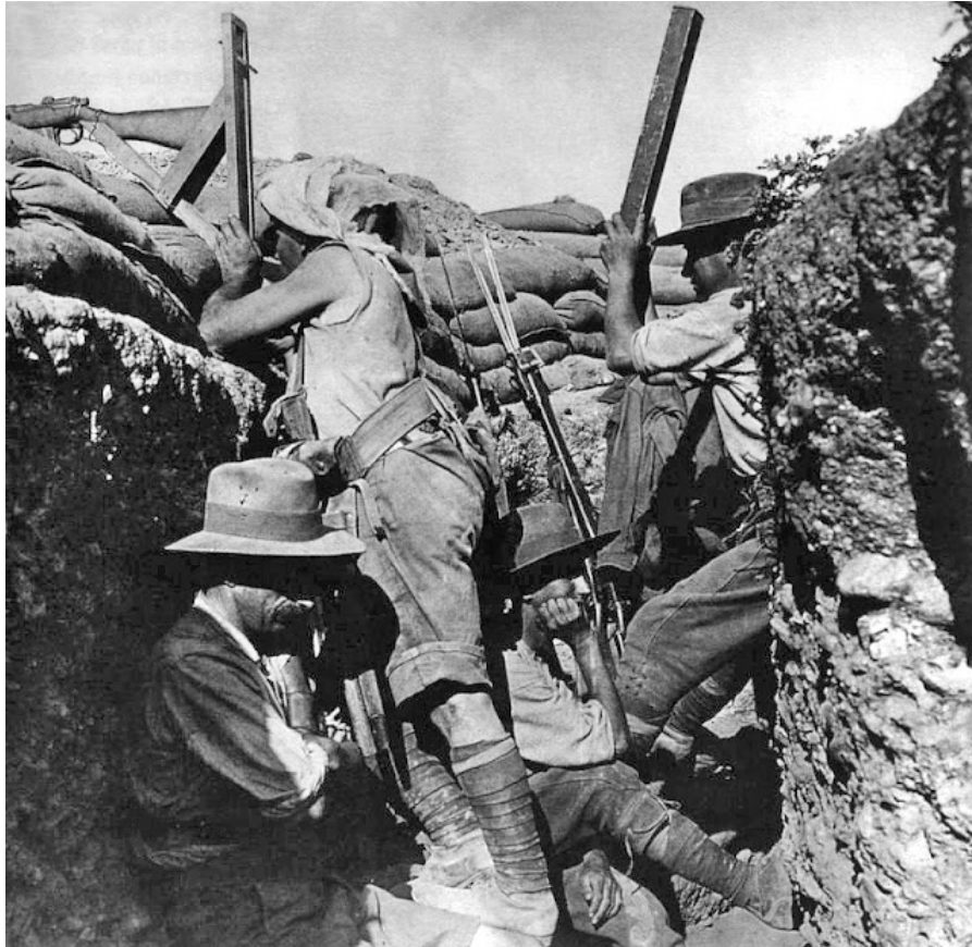
Source 42 The periscope rifle in Gallipoli 1915. An observer checks the results with a trench periscope. [ https://historicalphotosdaily.blogspot.com/2011/02/gallipoli-campaign-1915.html ]
