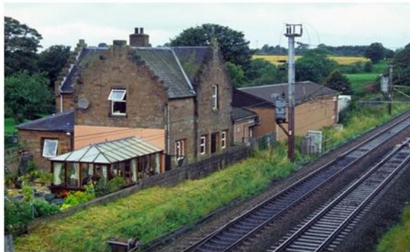
Former Caledonian Station, Gretna , now a private house
