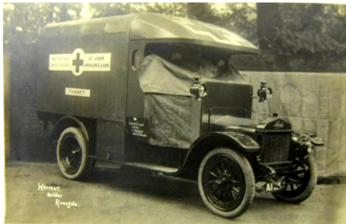
▲ The "Thanet" Ambulance before it went to France. The chassis was made by The Vulcan Motor & Engineering Co Ltd of Southport (Lancs) and the ambulance body was made Francis John Wraight, coachbuilder, whose works were at Eagle Hill, Ramsgate. The vehicle registration number is A1-RX (A1 was a London number and the RX might have signified 'Red Cross'). A different vehicle registration number would have been allocated to the vehicle when it went to France
