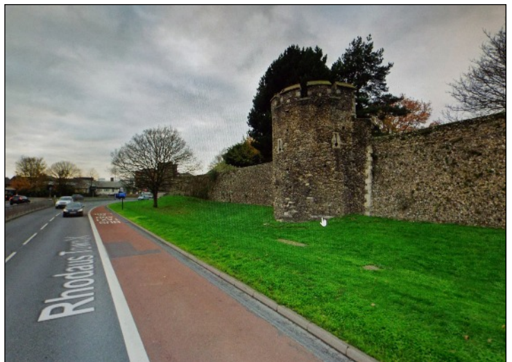
This image from Google Street View shows the same location today. The width of the Moat has been much reduced to accommodate the dual carriageway of which this stretch between Riding Gate and Pin Hill is known as Rhodaus Town
