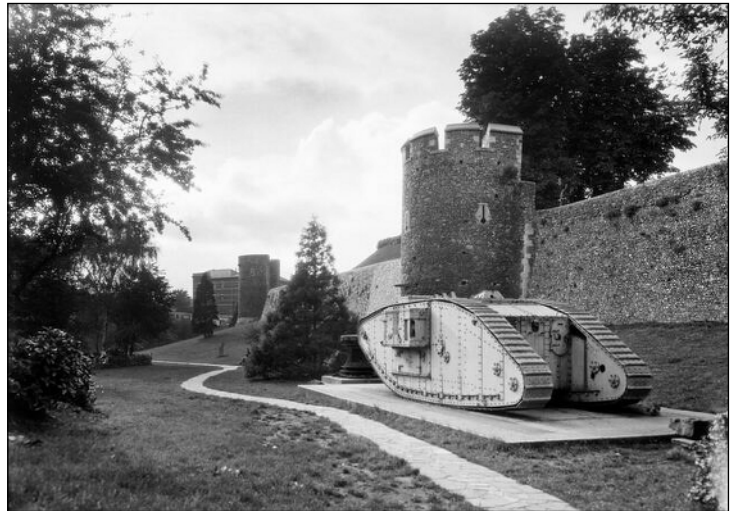
The above photo shows quite clearly where the Canterbury Tank was located in the Moat outside the city walls
