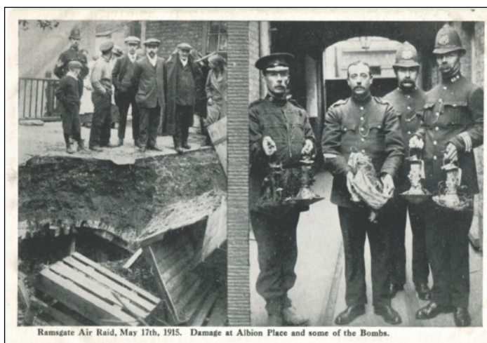
'Ramsgate Air Raid, May 17th, 1915. Damage at Albion Place and some of the Bombs.' (This particular air raid on Ramsgate is also covered by articles on pages 15 and 16 of this issue of Between the Lines - Ed.)
