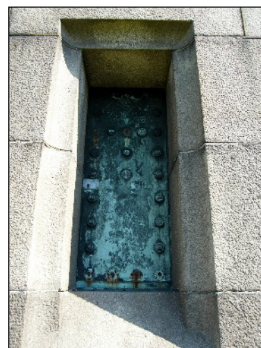
The locked doorway on the south-western side of the monument
